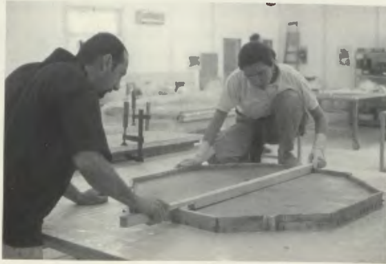
2. Application of mortar on a lightweight panel.
