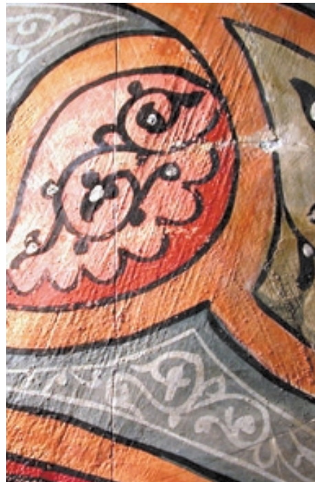
31. Dome 2. The surface roughness of the thin layer on the intonaco makes it appear to have been brushed on.
