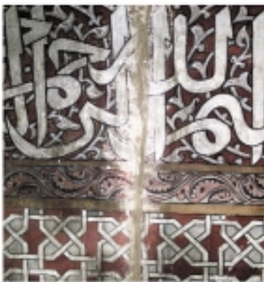
LOSSES IN THE COLOR DUE TO WATER INFILTRATION AND DEPOSITS OF MUD
