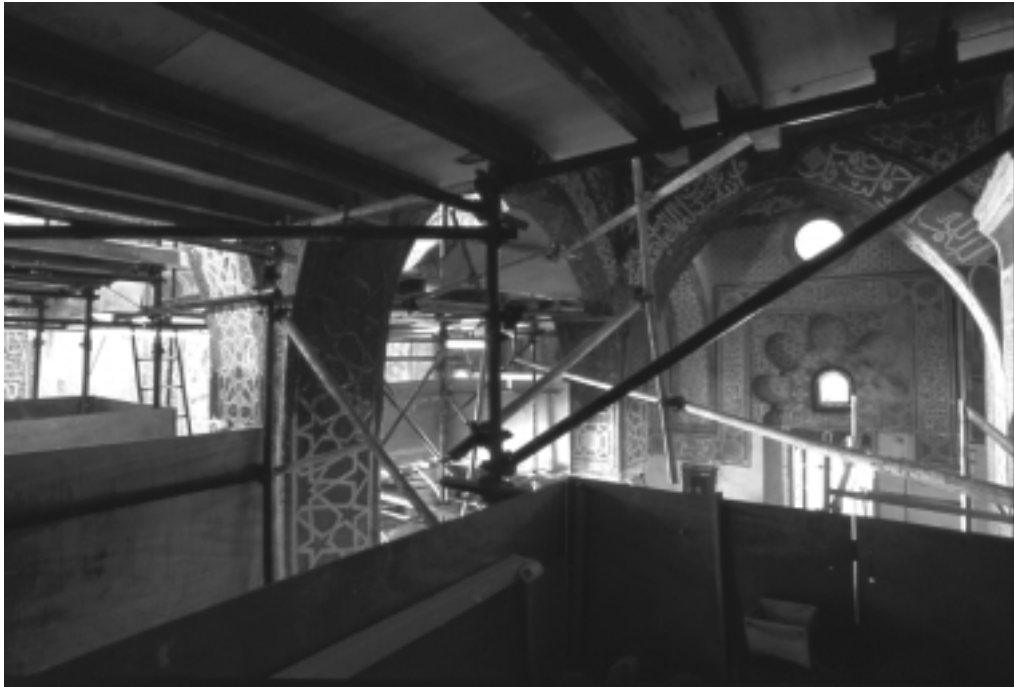
19 General view of the work-site with the scaffolding.
