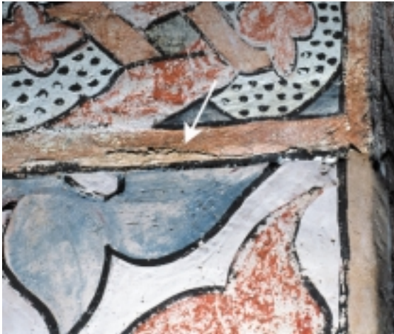
47. In dome 2 where the plaster had fallen we noted paint on the plaster surface partially covered by plaster from the surface below this level.
