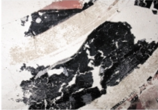
FLAKING OF COLOR AND DECOHESION OF THE INTONACHINO
