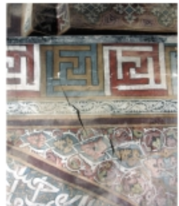
LOSSES IN THE PLASTER AND CRACKS
