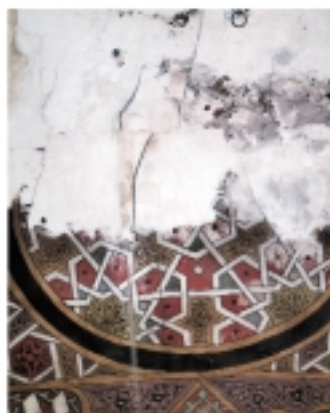
LOSSES IN THE PLASTER AND CRACKS
