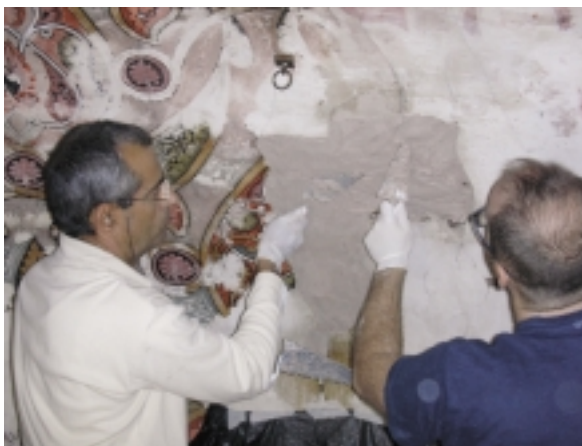
58. Filling of the lacunae of the intonaco with lime mortar.
