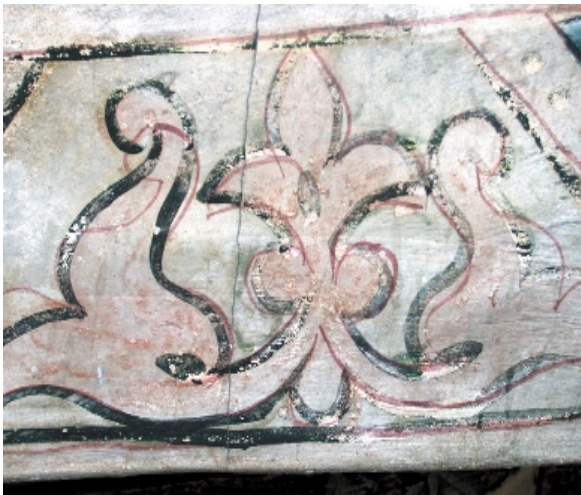
41. Dome 1. In areas where the original color is missing may be seen the preparatory drawings made with red ochre.
