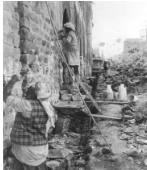
8. Restoration work began from the outside in.
