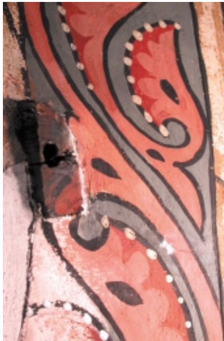
30. Dome 1. The face of the beams shows traces of painting done directly on the wood.
