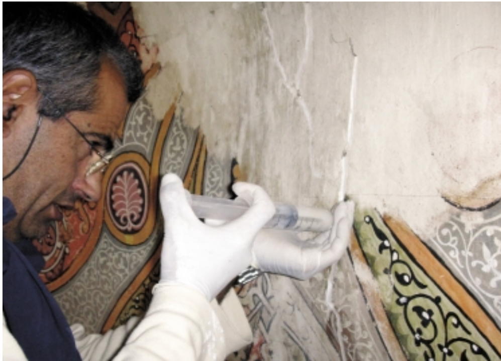
57 Consolidation of the detached plaster with injections of hydraulic consolidant.
