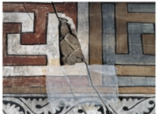
LOSSES IN THE PLASTER AND CRACKS
