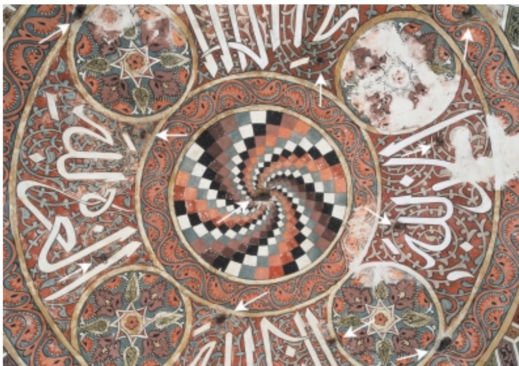
29. Dome 1. Detail showing 11 small wooden beams in situ.
