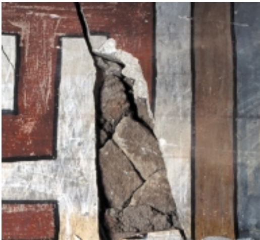
27. Dome 4. Stratigraphy of the support with the brick structure evident.
