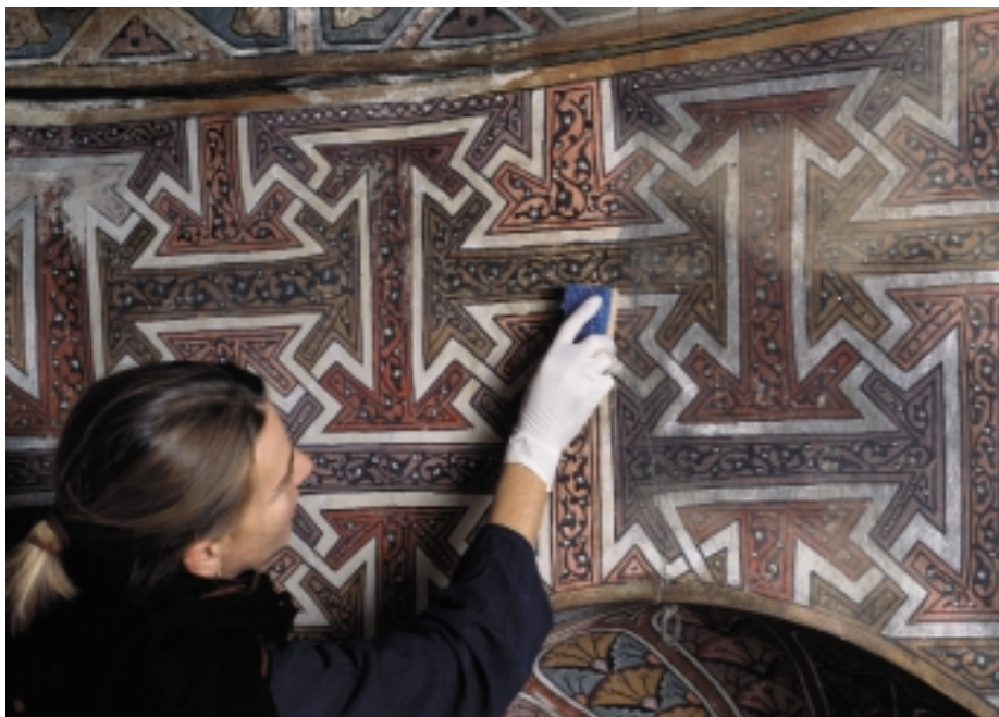
53 Cleaning of the coherent deposits with Wishab sponges.
