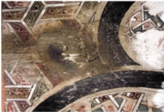
CARBONATE DEPOSITS
