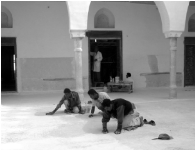
18. Polishing, or rather burnishing the surface of qudad with a smooth, rounded, riverine pebble produces an almost marble-like quality material
