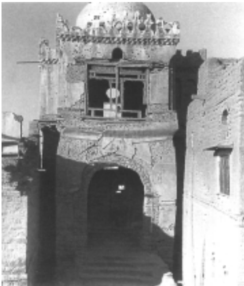
7. The project's real nightmare was the monumental eastern portal
