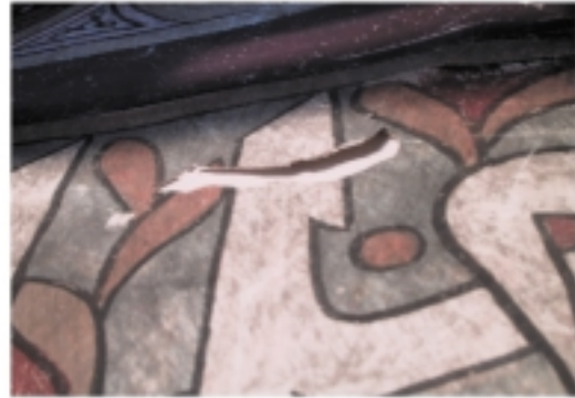
DETACHMENT OF INTONACHINO
