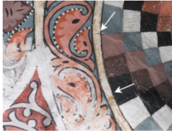
36. Dome 1. The mark left in the incisions are typical of those made in fresh plaster using a wooden stick
