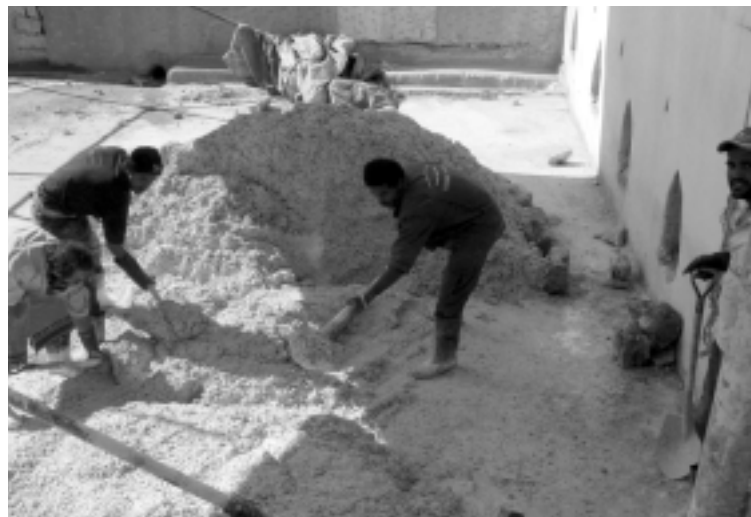
17. Pebbles and sand are mixed together in a ratio of two parts of aggregate to one part of lime. They are then blended together with water and pounded with a long shovel or wooden paddle.
