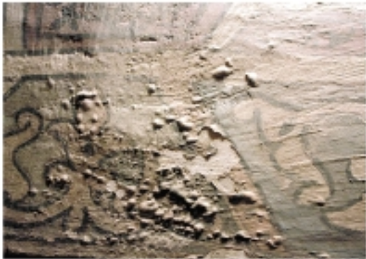
SUB-EFFLORESCENCES
