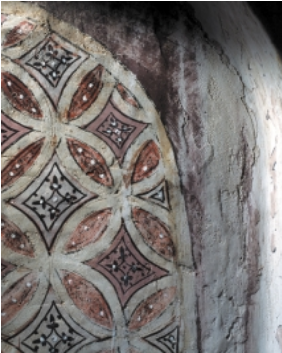
32. Dome 2. The blind niches show an overlapping of the intonaco which seems to be just a hasty fill, albeit subsequently painted
