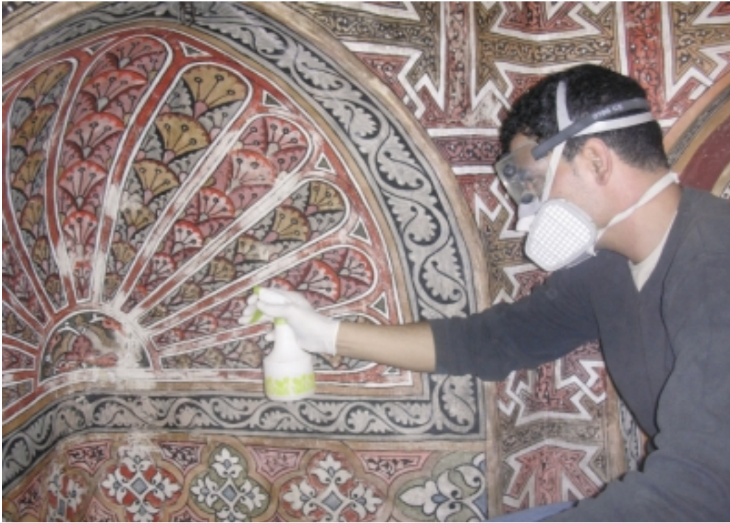
56 Consolidation of the pulverized colour with vaporized acrylic resin.
