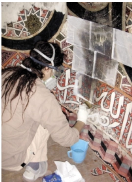
54 Chemical cleaning of the deposits of lampblack.
