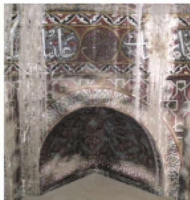
LOSSES IN THE COLOR DUE TO WATER INFILTRATION AND DEPOSITS OF MUD
