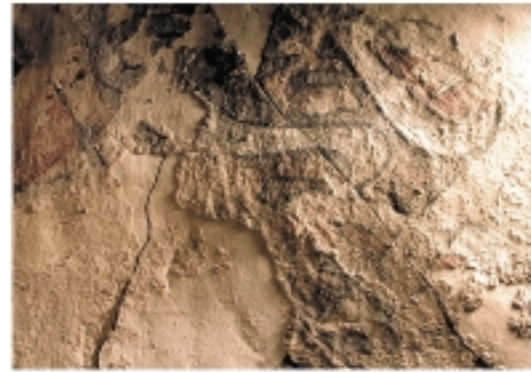
CRYSTALLIZATION OF SOLUBLE SALTS
