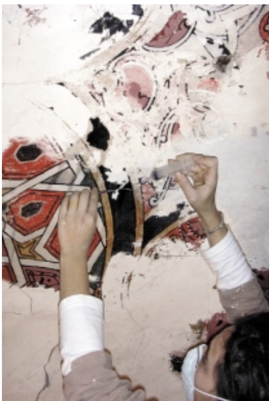
51 Consolidation of detached color from the surface of the plaster with infiltrations of acrylic resin.
