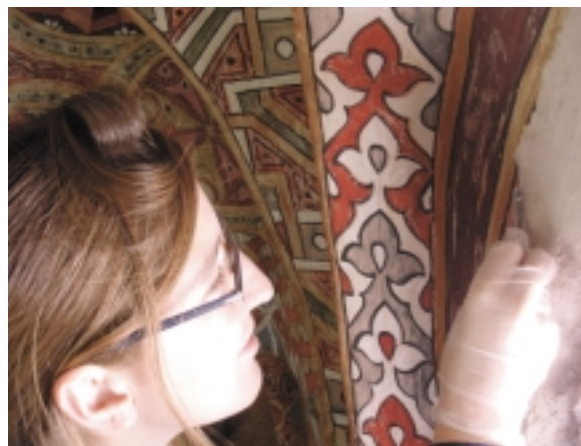
59. Filling of the fractures with gypsum based mortar.
